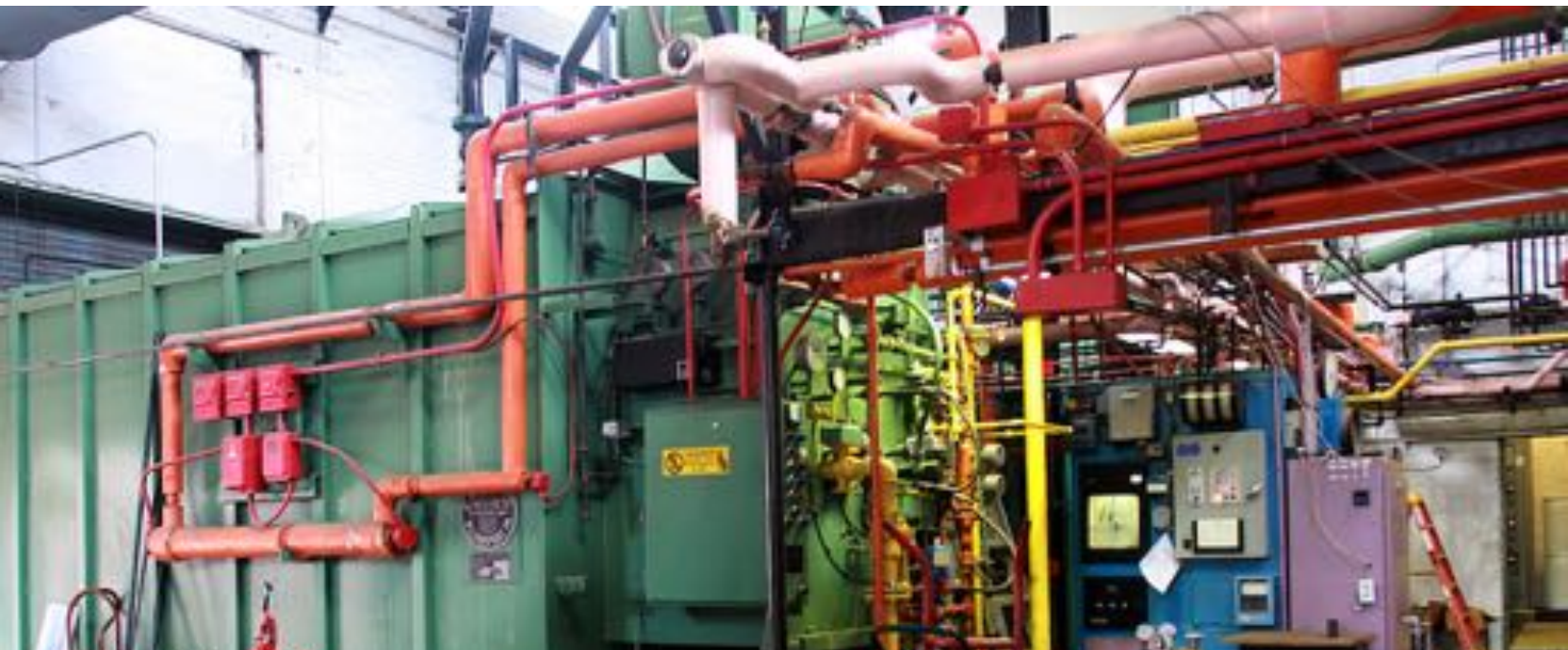
Saving energy in the heat plant with an expected payback period of 10 years.
